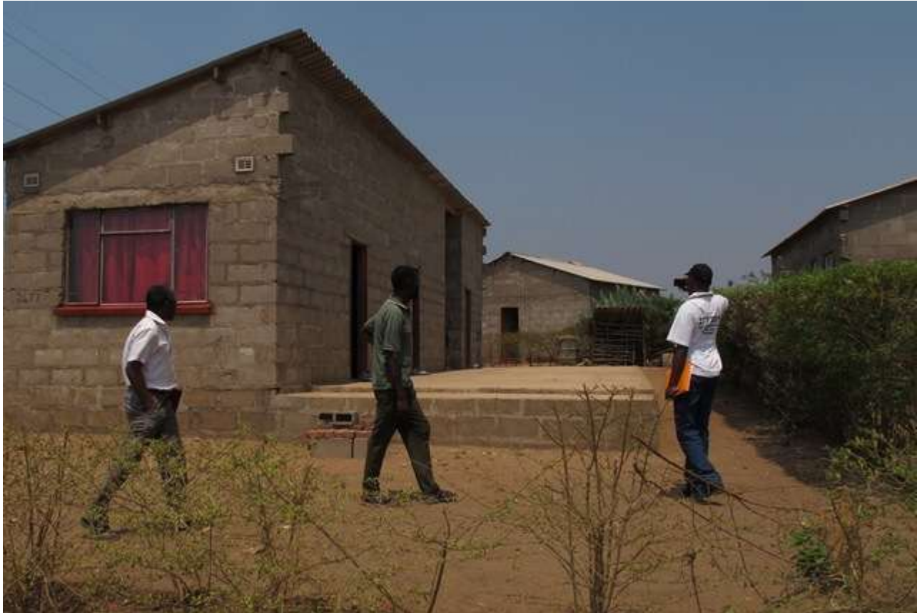
Half-built houses that are part of the Batonga Housing Co-operative in Kariba
