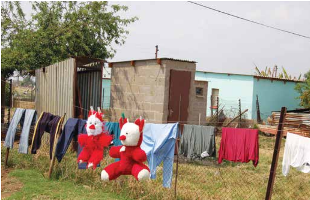
Figure 6: Newly constructed houses and toilets, Ndaka, KwaZulu-Natal
