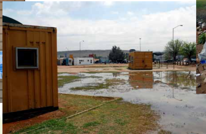
poorly maintained sewerage system
